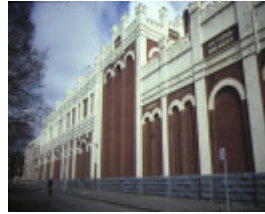
former victoria brewery victoria parade east melbourne front view sep 1985
