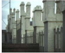
former victoria brewery victoria parade east melb detail of castellated style roof sep1985
