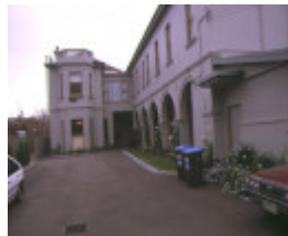
elizabeth house wellington prd east melb side view drive
