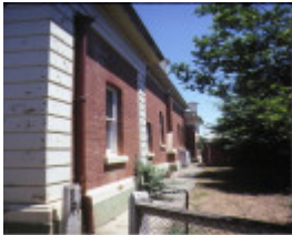
echuca court house side elevation dec1983
