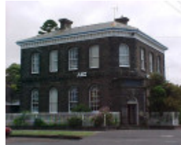
former bank of australasia sackville street port fairy front elevation nov1999
