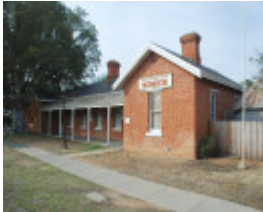
FORMER POLICE STATION SOHE 2008
