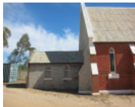
506-508 Napier Street, White Hills Uniting Church & Hall, vestry & possible early Methodist Church c1864 behind the later church
