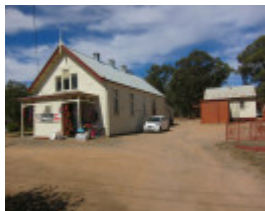
506-508 Napier Street, White Hills Uniting Church & Hall
