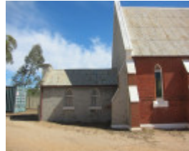
506-508 Napier Street, White Hills Uniting Church & Hall, vestry & possible early Methodist Church c1864 behind the later church
