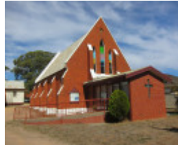
506-508 Napier Street, Uniting (former) Methodist Church with contemporary porch built in front
