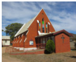
506-508 Napier Street, Uniting (former) Methodist Church with contemporary porch built in front
