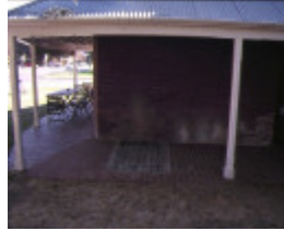
hopwood hotel echuca verandah
