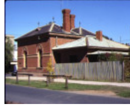
former customs house echuca side view
