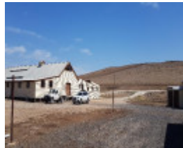
Greystones shearing shed 2019.jpg
