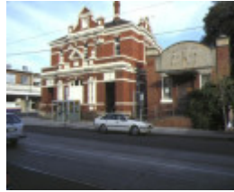
1 former elsternwick post office front view
