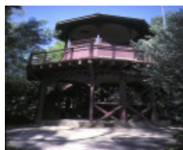
ripponlea elsternwick look out tower nov1984
