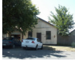
Shop (east shop of pair)
