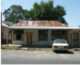
Shop (east shop of pair)
