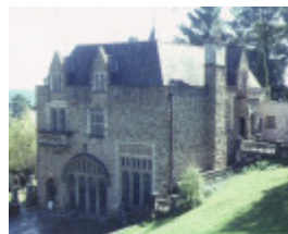
montsalvat hillcrest avenue eltham view of windows
