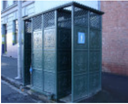
Urinal Queensberry & Elizabeth St exterior KJ 21 06 2007
