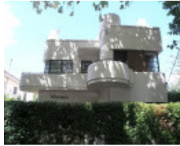
WINDERMERE FLATS SOHE 2008
