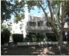
WINDERMERE FLATS SOHE 2008
