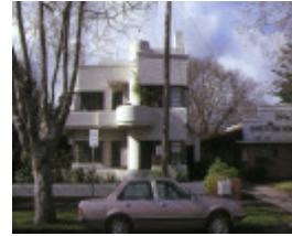
1 windermere flats broadway elwood front elevation jul1989
