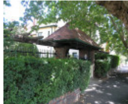
HARTPURY COURT COMPLEX SOHE 2008
