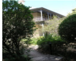
HARTPURY COURT COMPLEX SOHE 2008
