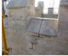
Before Photograph - Reference F3866 2014
