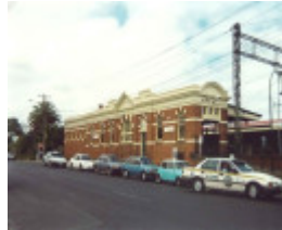
Caulfield Railway Station platform 4, August 1995
