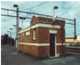
Caulfield Railway Station stores building, August 1995
