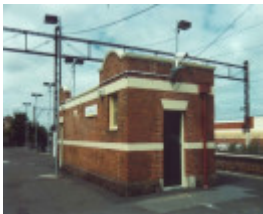
Caulfield Railway Station stores building, August 1995
