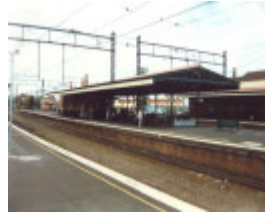
Caulfield Railway Station platform 2 and 3, August 1995
