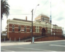
Caulfield Railway Station, platform 1, August 1995
