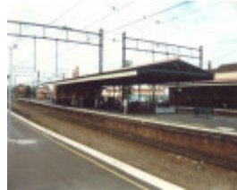
Caulfield Railway Station platform 2 and 3, August 1995
