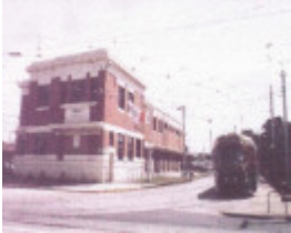
Glen Huntly Tram depot, Glen Huntly Rd Caulfield
