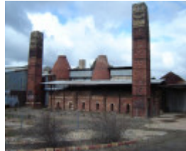
1 Bendigo Pottery North West Facade and Rectangular Kiln 2 (S9), Bottle Kilns 3 & 4 (S3 & S4) and Chimneys 1, 2 & 3 (S10, S11 & S12) 16 August 2005 mz
