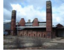
1 Bendigo Pottery North West Facade and Rectangular Kiln 2 (S9), Bottle Kilns 3 & 4 (S3 & S4) and Chimneys 1, 2 & 3 (S10,S11 & S12)16 August 2005 mz
