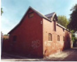
Stables, 8 Park Crescent Caulfield, August 2000
