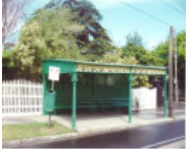
Tram Shelter Corner Balaclava & Orrong Roads Caulfield
