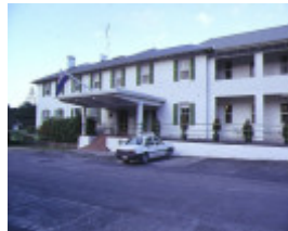
1 erskine house mountjoy parade lorne front view
