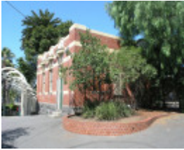
ESSENDON RAILWAY STATION COMPLEX SOHE 2008
