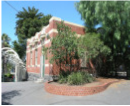
ESSENDON RAILWAY STATION COMPLEX SOHE 2008
