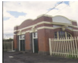
essendon railway station complex buckley street essendon store building oct1998
