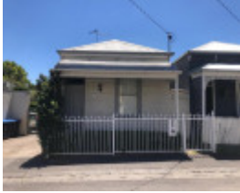
1 Bayview Street, Prahran
