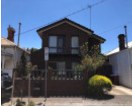
19 Bayview Street, Prahran
