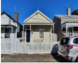
24 Bayview Street, Prahran
