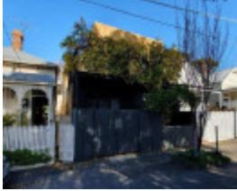
28 Bayview Street, Prahran
