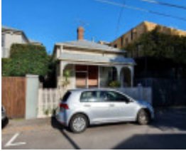
30 Bayview Street, Prahran
