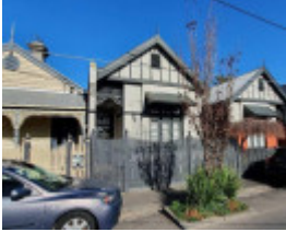
42 Bayview Street, Prahran
