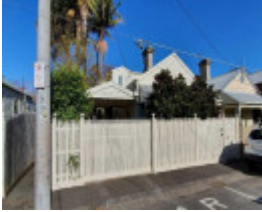
56 Bayview Street, Prahran
