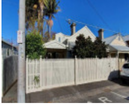
56 Bayview Street, Prahran
