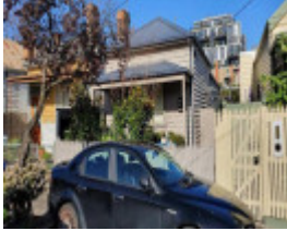
72 Bayview Street, Prahran
