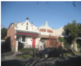
Terrace at 8-12 Lorne Road.
