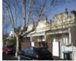
Victorian terrace on Mt Pleasant Grove
