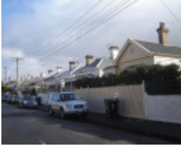
Victorian workers cottages on the north side New Street.
