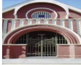
euroa courthouse detail of entrance
