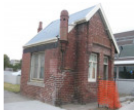
Former Ferry Terra Cotta & enamel brickworks office albert Street brunswick from the northwest
