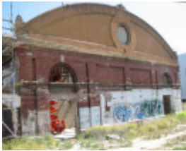
FORMER BRUNSWICK GAS & COKE COMPANY RETORT HOUSE SOHE 2008
