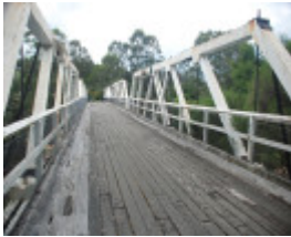
TIMBER TRUSS AND CONCRETE BRIDGE SOHE 2008
