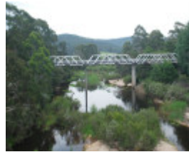
TIMBER TRUSS AND CONCRETE BRIDGE SOHE 2008
