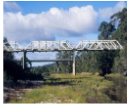
h01214 1 timber truss and concrete bridge over genoa river genoa western side she project 2003
