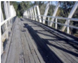
h01214 timber truss and concrete bridge over genoa river genoa decking she project 2003
