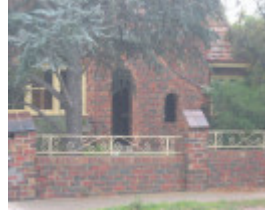
18 Barton Street, Fence
