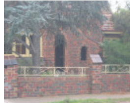
18 Barton Street, Fence
