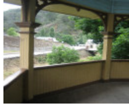
Walhalla Bandstand looking towards stone wall
