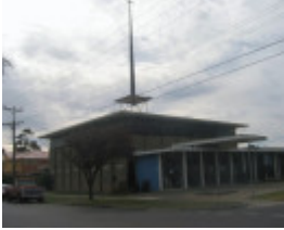
St George's Church, 32-34 Ralph Street
