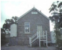
faraday primary school no 797 calder highway faraday front view aug 84
