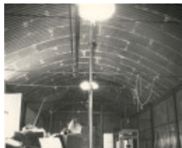
Porter prefabricated iron store
