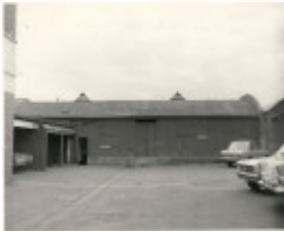
Porter prefabricated iron store
