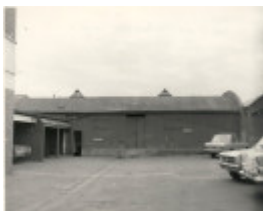
Porter prefabricated iron store
