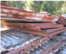
Porter prefabricated iron store
