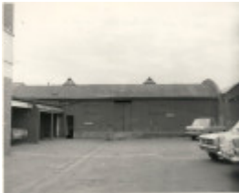
Porter prefabricated iron store
