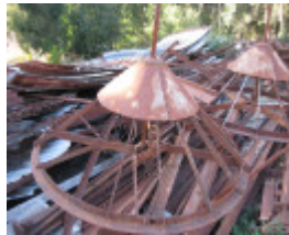
Porter prefabricated iron store
