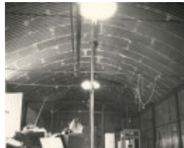
Porter prefabricated iron store
