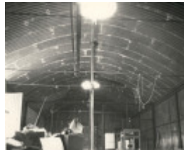
Porter prefabricated iron store
