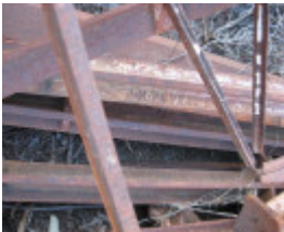
Porter prefabricated iron store
