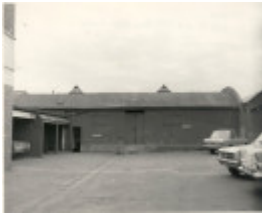
Porter prefabricated iron store
