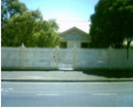
158 Aberdeen Street, Geelong West
