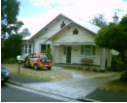
24 Lupton Street, Geelong West
