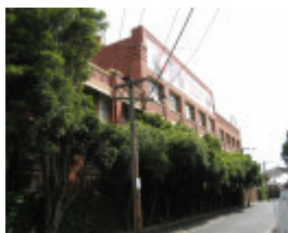
Former Wertheim factory Richmond_north wing incl Heinz additions_Feb 08
