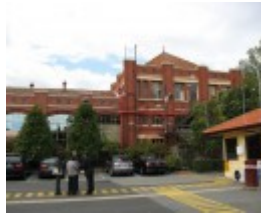
Former Wertheim Factory Richmond_southern elevation of east wing_Feb 08
