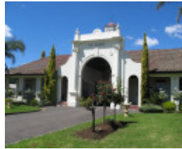
Beam Wireless Receiving Station Mt Cottrell recreation bldg
