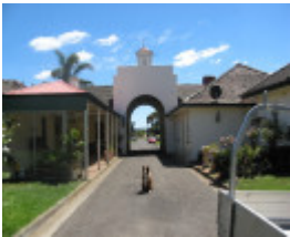
Beam Wireless Receiving Station Mt Cottrell rear of recreation bldg
