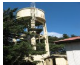
Concrete water tower
