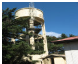
Concrete water tower
