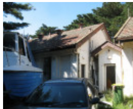
Beam Wireless Receiving Station Mt Cottrell porch between 2 operations bldgs
