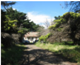
Beam Wireless Receiving Station Mt Cottrell operations bldgs
