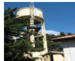
Concrete water tower
