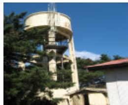
Concrete water tower
