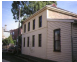
former national school bell street fitzroy building 2 1994
