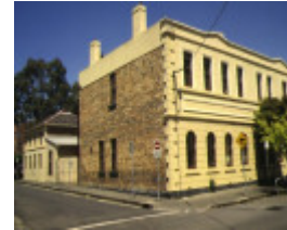
former national school bell street fitzroy front corner view dec1994
