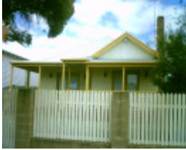
31 Lupton Street, Geelong West
