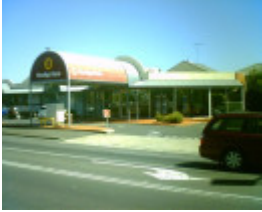
62a - (Unit 2) Aberdeen Street, Geelong West
